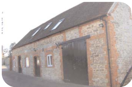
Clay tile, stone with brick dressings Stables, [Archangel House (The Old Vicarage)] the Vicarage
