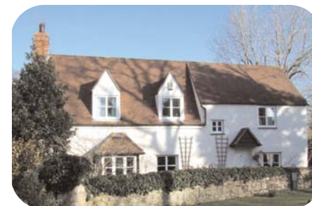
Steeply pitched dormers 90 (Mosses House [Cottage]) Appleton Road
