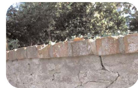
Stone wall with brick capping, [Archangel House (The Old Vicarage)] The Vicarage
