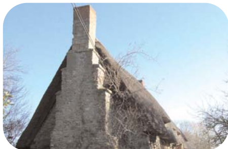
Stepped stone chimney stack 41 Leys Road
