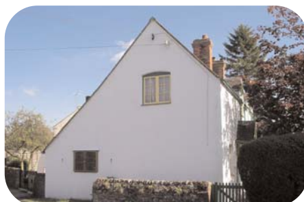
Raking roofed outshot No11 Appleton Road
