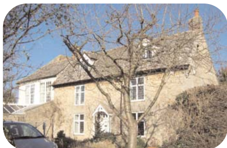
Wood mullioned and transomed windows with leaded lights, Cutts End Cottage
