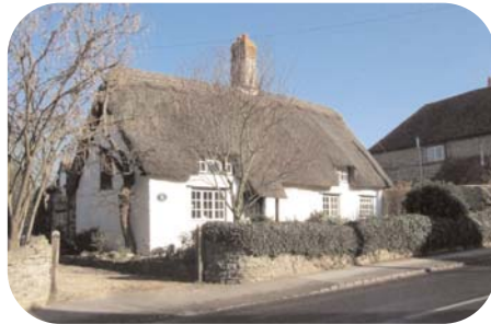
Thatched roof and painted stonework, 6 High Street (Stonehaven Cottage)
